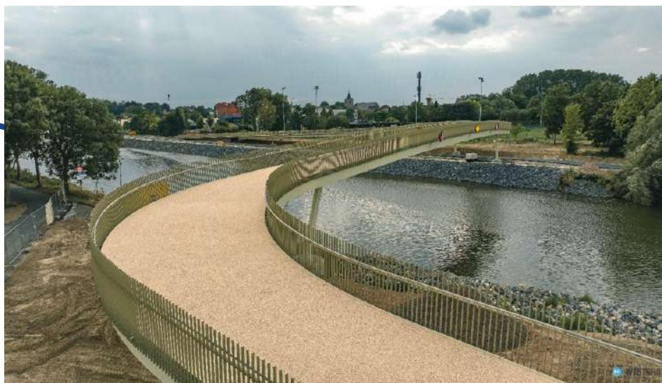
The De Blauwersbrug cycling bridge in Menen, Flanders, inaugurated in August 2025 (Photo credit: © De Vlaamse Waterweg nv)
