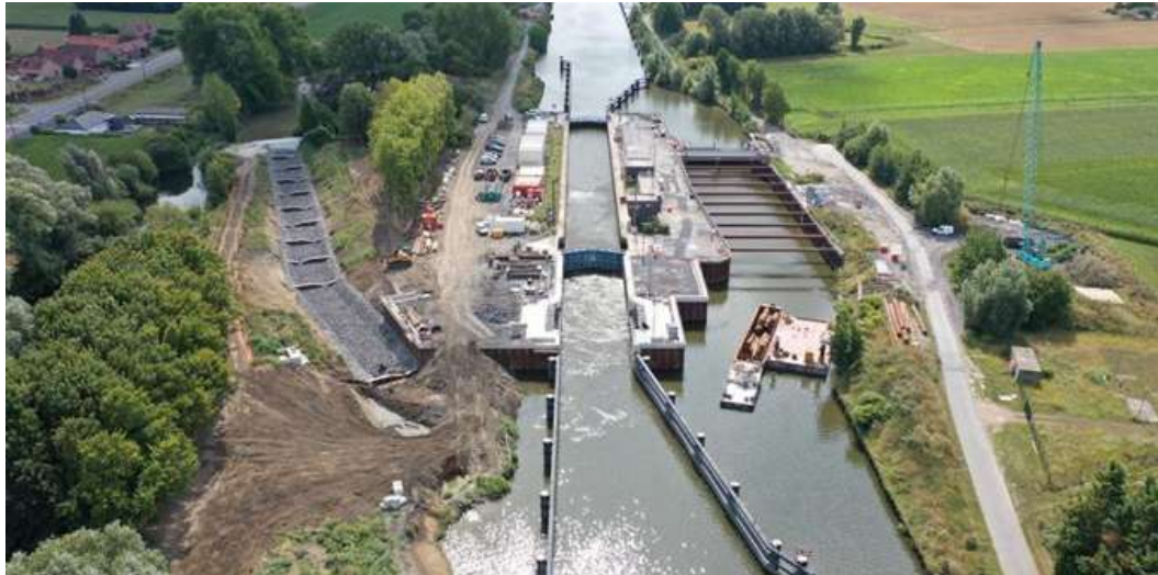
Extension of the Quesnoy-sur-Deûle lock in 2025 (Photo credit: © INGENO)
