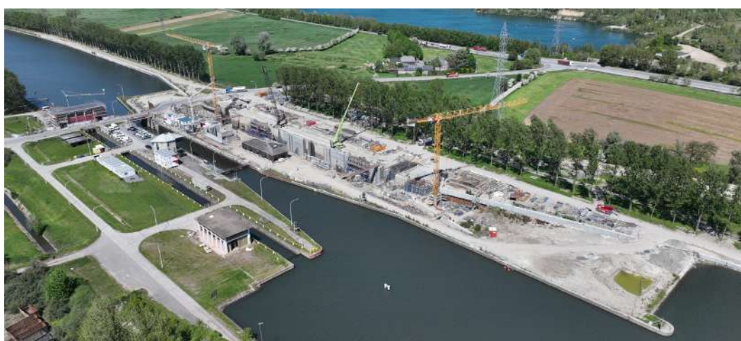
Modernisation of the Obourg lock complex on the Centre Canal, Wallonia (Photo credit: © SPW)
