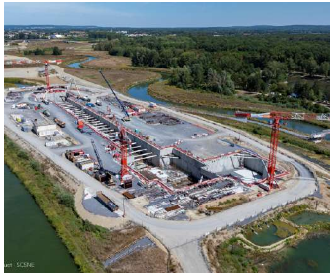
Construction site of the Montmacq-Cambronne-lès-Ribécourt lock in the Oise (Photo credit: © SCSNE – Odile and Jean-Christophe Hecquet)
