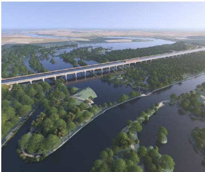
The Somme Canal Bridge (Photo credit: © Canaleau Lavigne Chéron Architectes)
