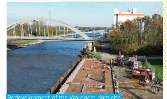
Redevelopment of the Waregem dam site
