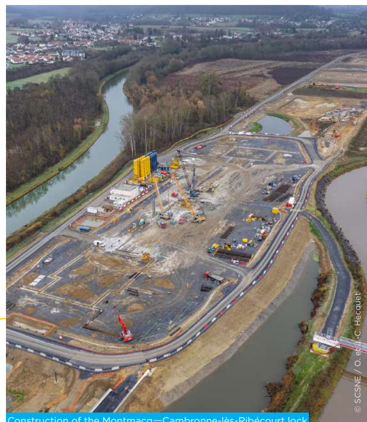
Construction of the Montmacq—Cambronne-lès-Ribécourt lock
