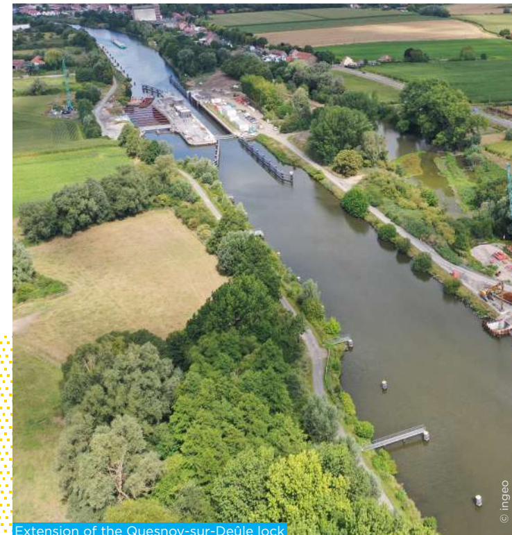
Extension of the Quesnoy-sur-Deûle lock
