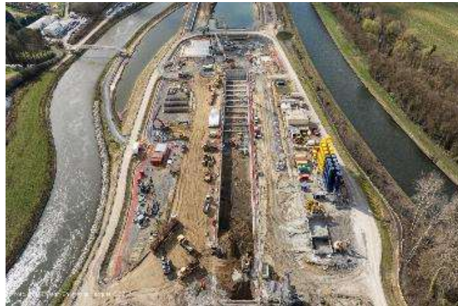
Construction work on the Montmacq lock (CSNE) April 2026
