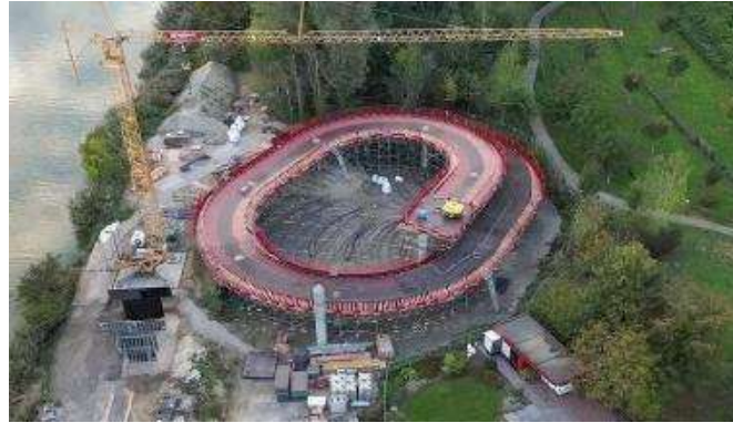
Construction work on the Ingelmunster bridge (Flanders)
