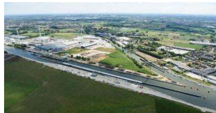
Construction works on the new Sint-Baafs-Vijve lock (2023 – crédits : @DVW)
