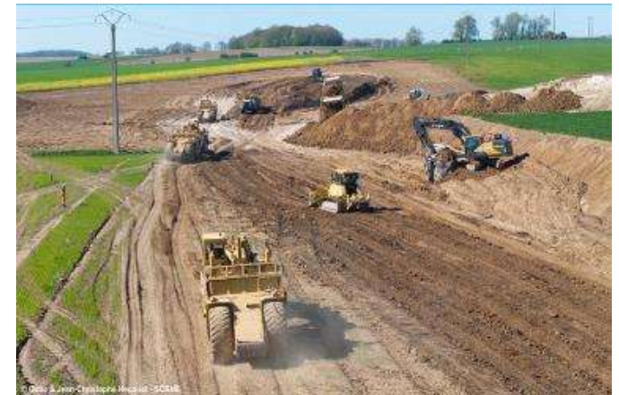
Earthworks of the Oisy-le-Verger lock (CSNE) June 2026
