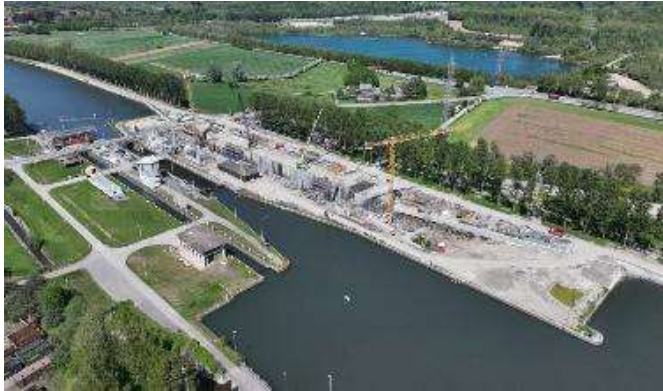
Construction work on the new lock of Obourg (Wallonia)
