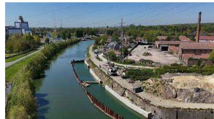
Development work on the Nimy Blaton canal (Wallonia)
