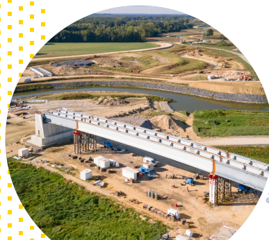
RD66 bridge at Montmacq - Cambronne-lès-Ribécourt
