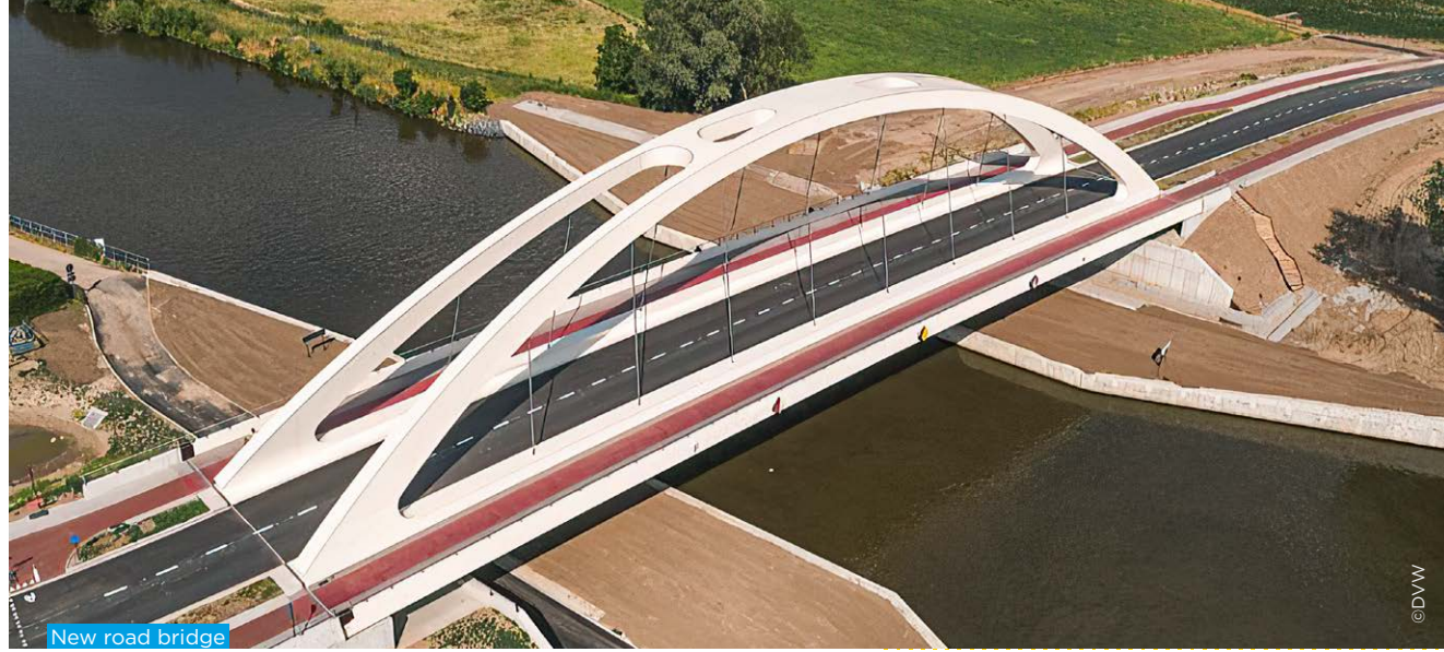
New road bridge between Bissegem and Marke
