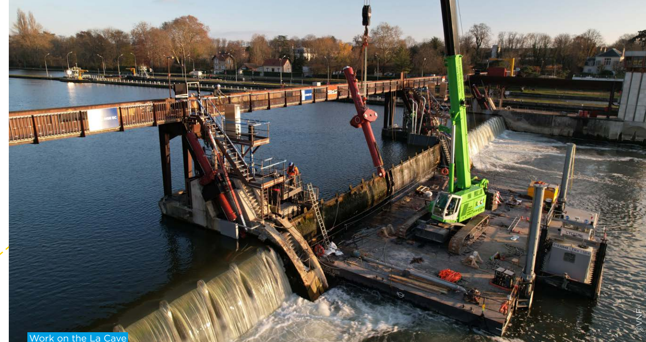
Work on the La Cave dam
