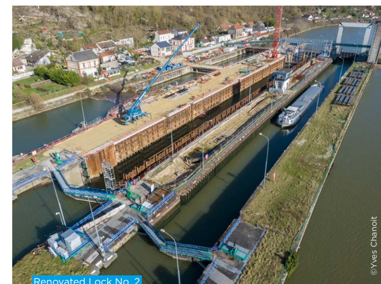
Renovated Lock No. 2 at Méricourt
