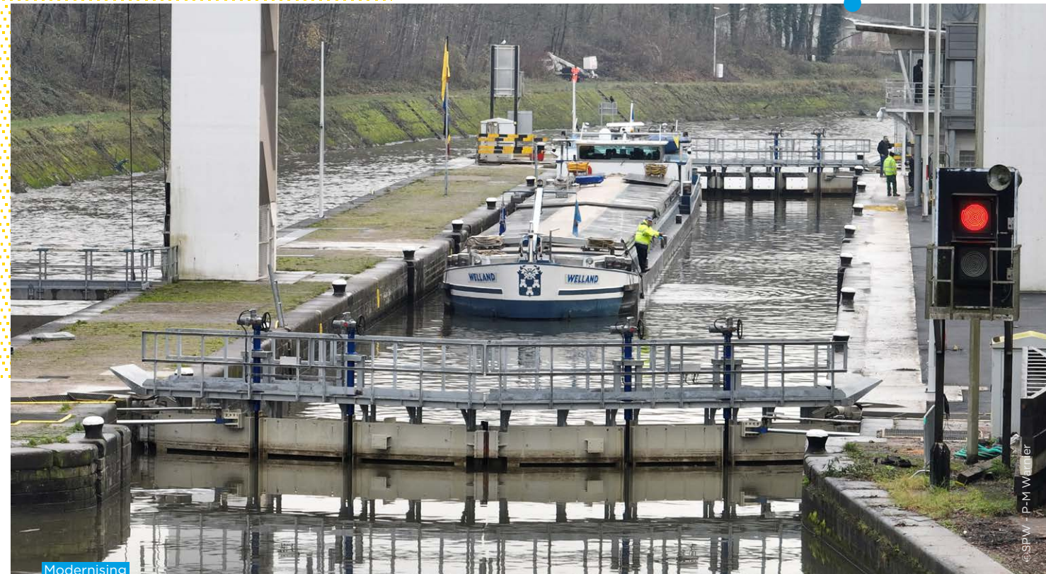
Modernising Auvelais lock
