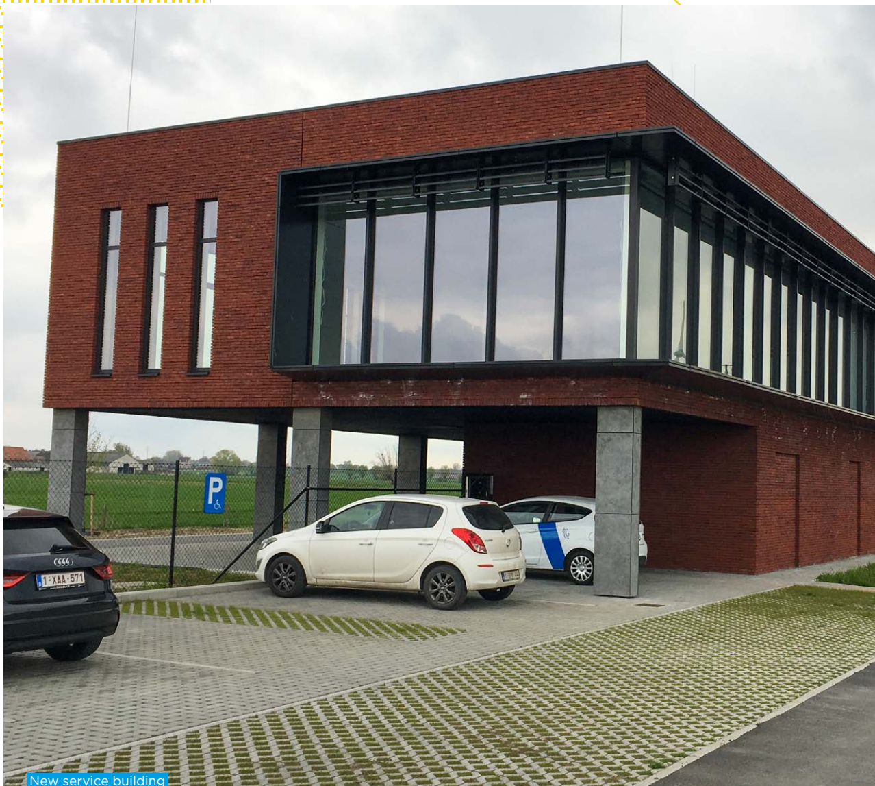
New service building at the Vive-Saint-Bavon lock
