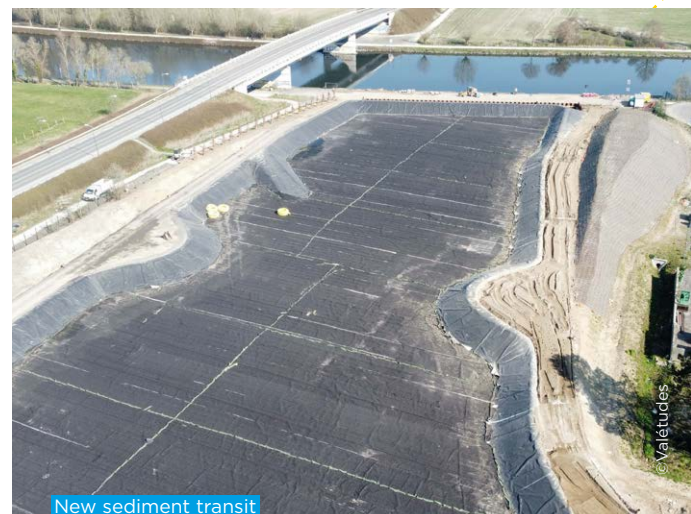
New sediment transit and drying platform in Wambrechies
