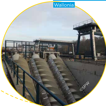
Lift station on the Charleroi-Brussels canal, Wallonia
