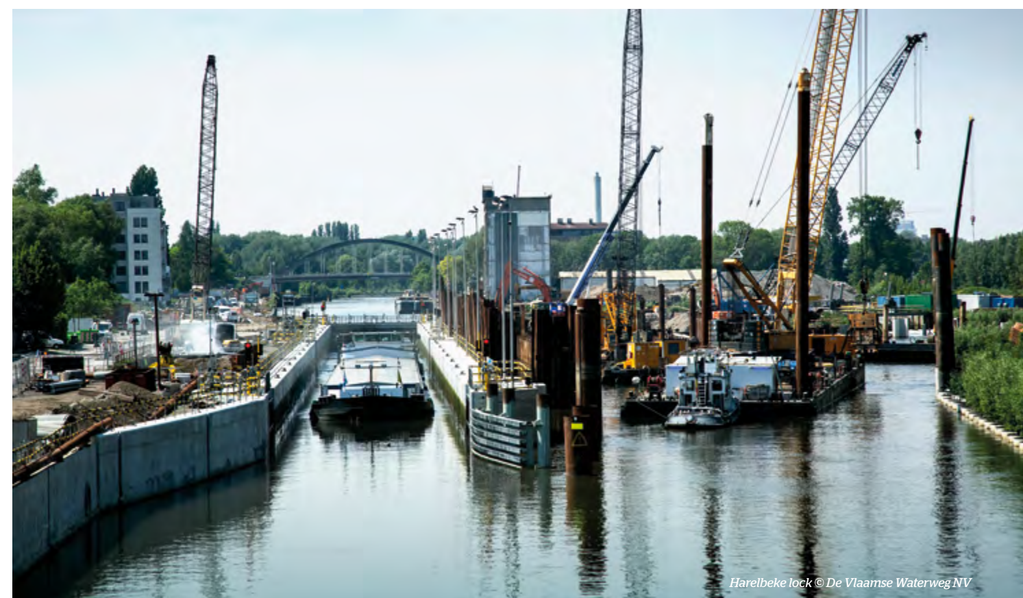
Locked gate replacement at Les Fontinettes © VNF
