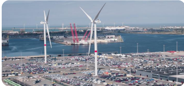
Energy locally produced and stored
